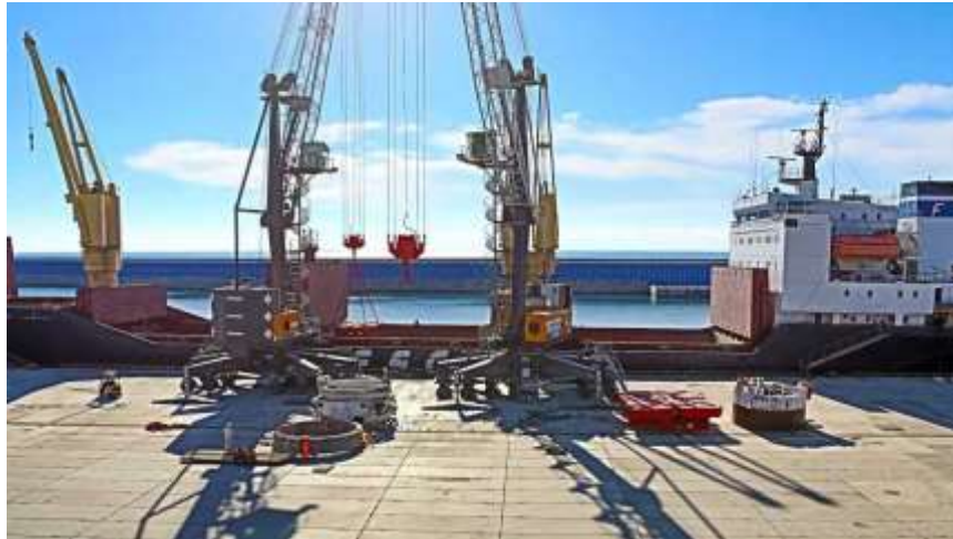
Figure 3 – Loading operations by mobile crane
