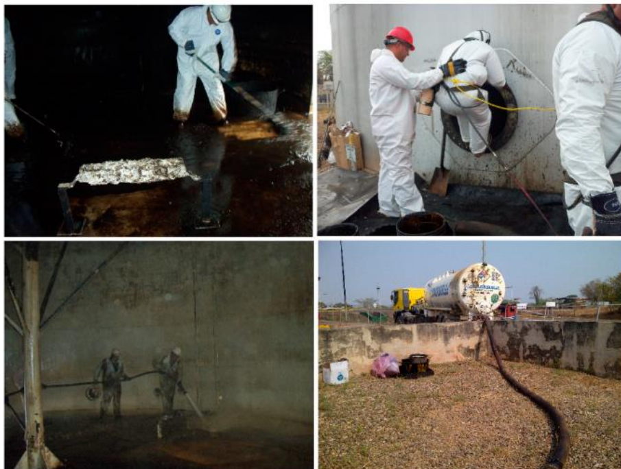
Fig. 1 The process of cleaning a surface contaminated with oil products by cryogenic blasting.
