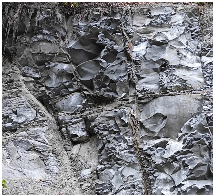
Figure 3. Fracture system with tectonic breccia in tuffs of the Middle Badenian Teresva Formation. Solotvine Basin, northwestern outskirts of village Lazy.
