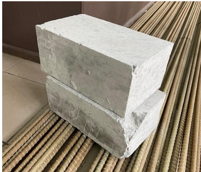
Figure 1. Cut out fragments of concrete from a slab with fiberglass reinforcement inside (from the central section of road slab).
