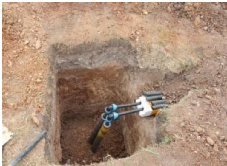
Figure 3. Schematic diagram of the U-shaped underground heat exchanger and its connection to the central manifold.
