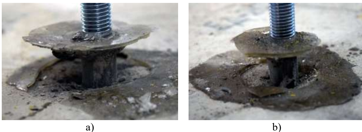
Figure 2. Failure modes of epoxy bonded anchors in cells P3V3 (a) and P4V3 (b) after pull-out tests
